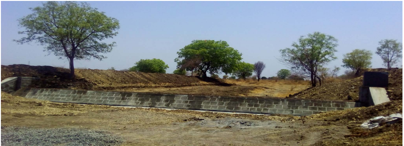
Check-dam construction under watershed management in Bothali, Wardha district, Maharashtra
